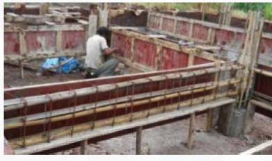
Bamboo reinforcement in plinth beams
