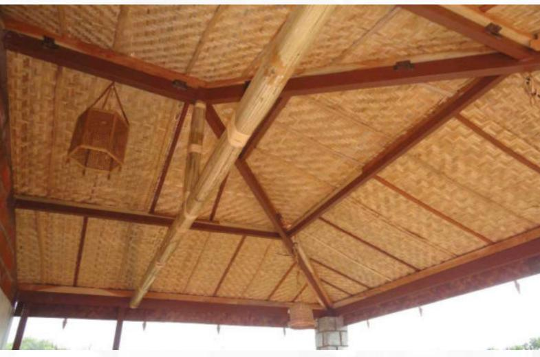
Bamboo as a roofing material
